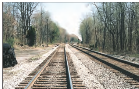
The railroad tracks near Bucklodge.
