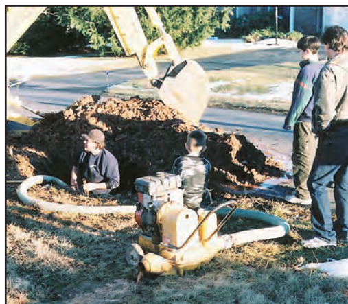
Poolesville boys supervise town workers repairing a water main break.
