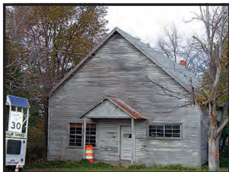
The Barnesville Town Hall, With Work Yet To Be Done
