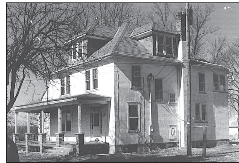
Original King farmhouse just prior to demolition.
