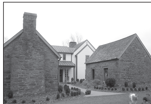
A detached kitchen (right) was an early fire protection idea.
